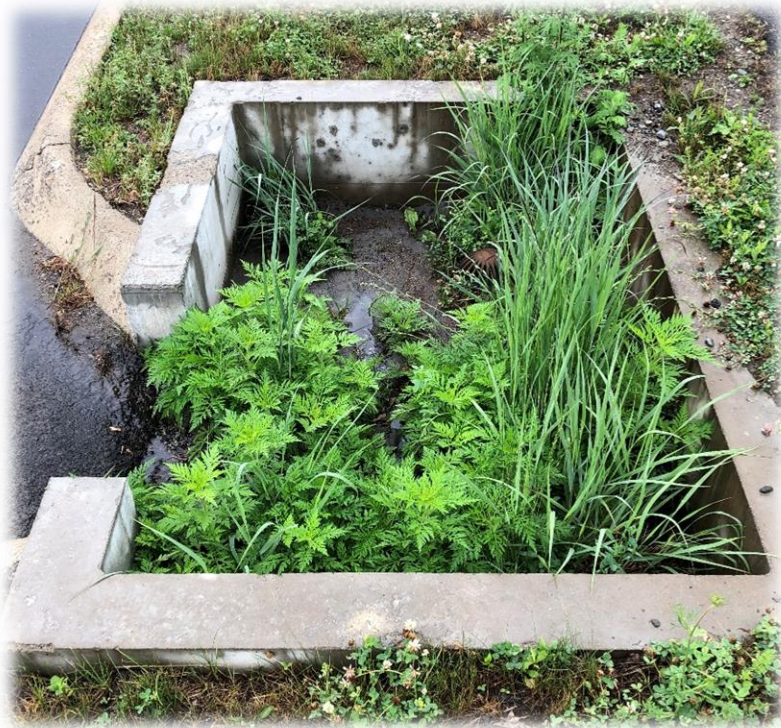
Orono roundabout stormwater planter
